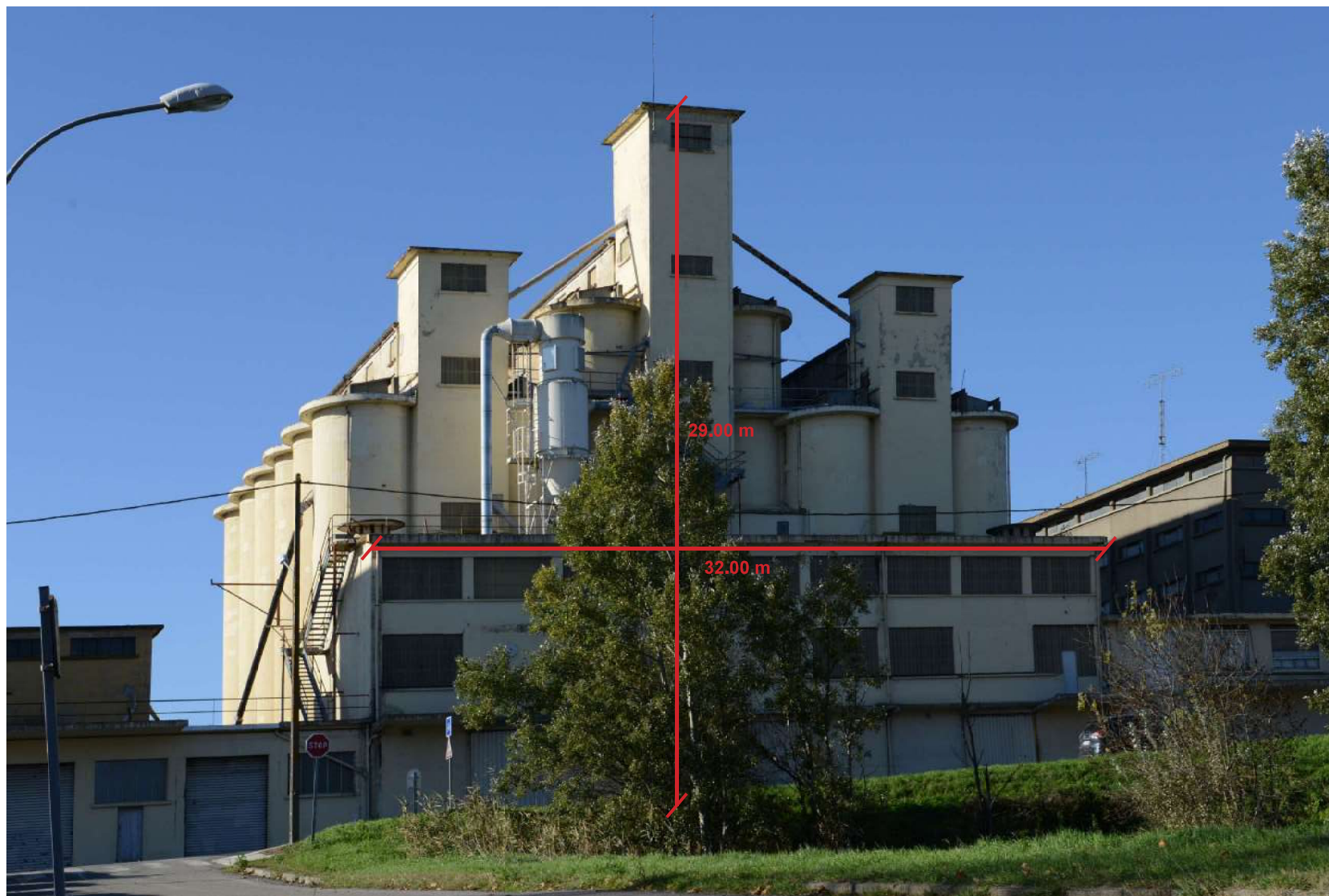
Silos 1930 (Dimensions approximatives)
